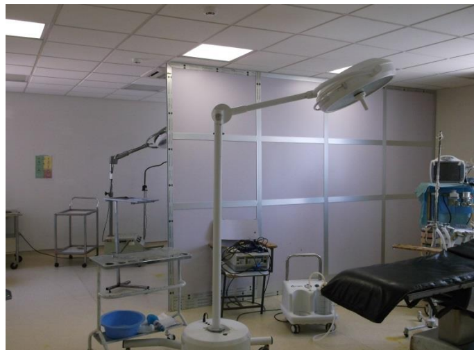
The new OR dividing wall at Felege Hiwot, Bahir Dar
